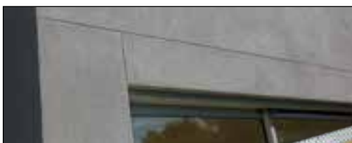
Figure 3.4.1 Neat finish of horizontal joints
