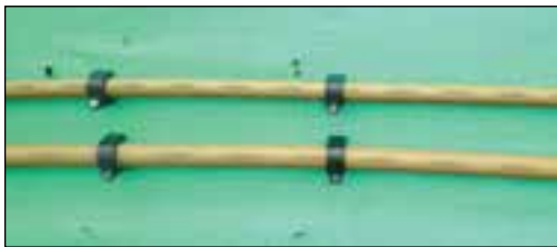
Figure 3.3.1 Installed piping services prior to the installation of Hebel PowerPanel XL
