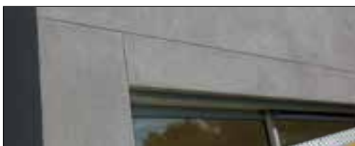
Figure 3.4.1 Neat finish of horizontal joints
