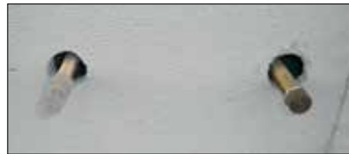
Figure 3.3.2 Neat finishes of installed services
