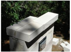
The capping blocks are laid flat and can overhang the front and rear of the wall for a great feature.
