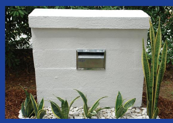
This project is easily constructed in a few hours and is built on an existing or purpose laid concrete footing that has a minimum surface area of 1000mm x 300mm.
