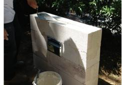
The fifth course is to "cap" the wall and cover the cavity between the front and rear walls.
