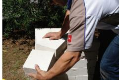
Cut 2 blocks to the width of the wall, and place these blocks at each end of the 3rd course as shown.
