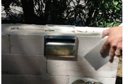
Fill the remaining 3rd course by cutting blocks to the required size to suit the gap either side of the letterbox. Use Hebel Adhesive on all block joins.
