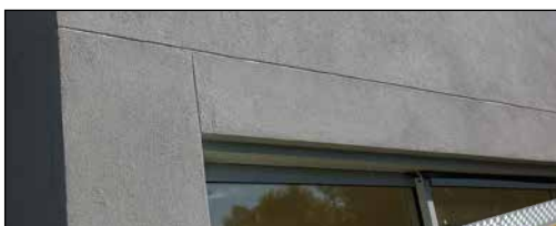
Figure 3.4.1 Neat finish of horizontal joints
