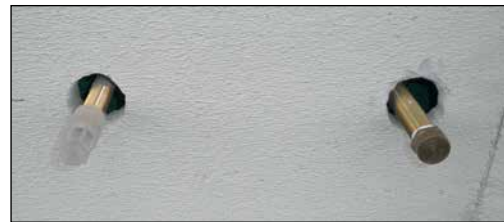
Figure 3.3.2 Neat finishes of installed services
