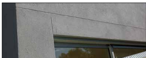
Figure 2.7.1 Neat finish of horizontal joints
