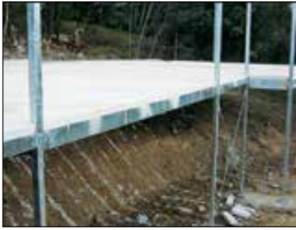
Fig 1.1.1 Residential Suspended Ground Floors
