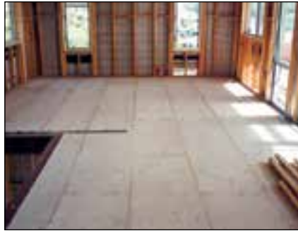
Fig 1.1.2 Residential Suspended First Floors
