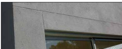
Figure 2.7.1 Neat finish of horizontal joints
