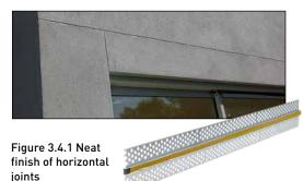
The external aluminium render bead can be used as an option at horizontal joints to provide neat and consistent finish joints. After installation of the PowerPanel<sup>XL</sup> panels, the render bead is applied and hold onto place by using Hebel adhesive. Suitable external grade sealant is to be applied at the joint before rendering.
