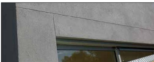
Figure 3.4.1 Neat finish of horizontal joints
