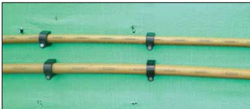
Figure 3.3.1 Installed piping services prior to the installation of Hebel PowerPanel<sup>XL</sup>
