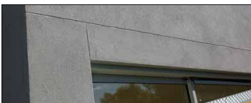
Figure 3.4.1 Neat finish of horizontal joints
